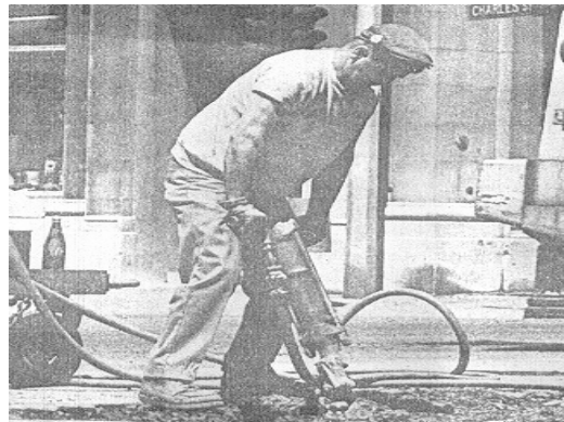
Man working with a jackhammer.
