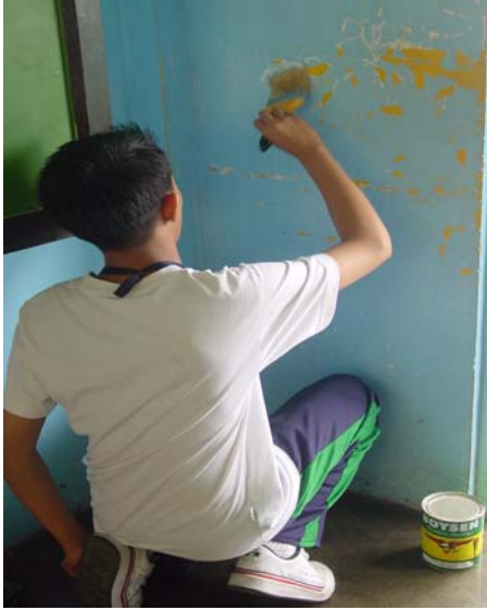
Painting the wall of a room
